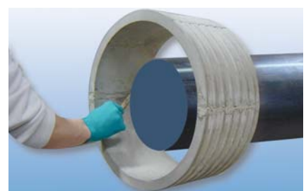
Distribute filler evenly so that the inner surface forms a homogeneous seal surface, smooth with emery cloth, if necessary.
