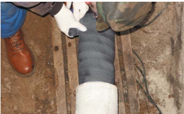
3. After saturating with water, wind the Pipecast tape around the pipe with a minimum of 1 x 75% (4 layers) overlap.
