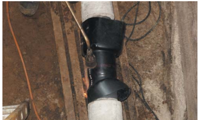
2. Installing the shrink sleeve
