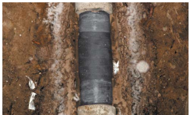
6. Pipecast after application.
