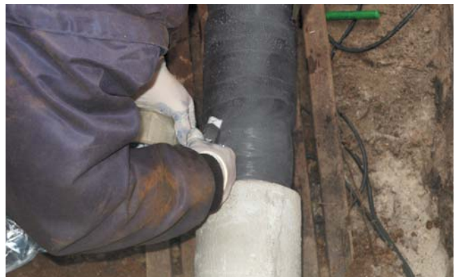
4. Wind adhesive tape around the ends of the Pipecast tape in order to press it firmly on to the pipe.
