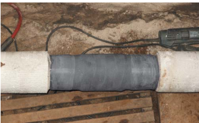
5. Allow the Pipecast to cure for 20-30 minutes at 23°C. It is ready to be buried after in approx. 1 hour.
