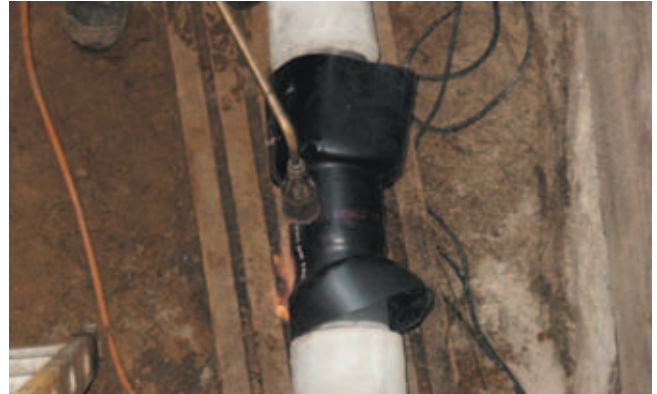
2. Installing the shrink sleeve
