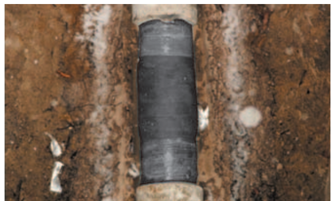
6. Pipecast after application.
