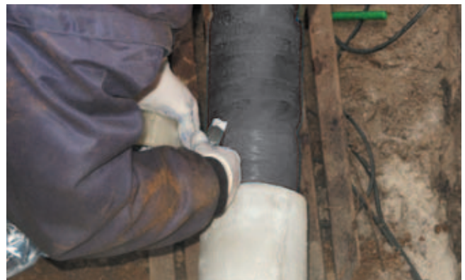
4. Wind adhesive tape around the ends of the Pipecast tape in order to press it firmly on to the pipe.
